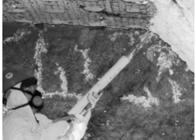
Foamfrax Installation
